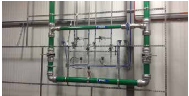
Inert gas Transair® 3" (76 mm)
