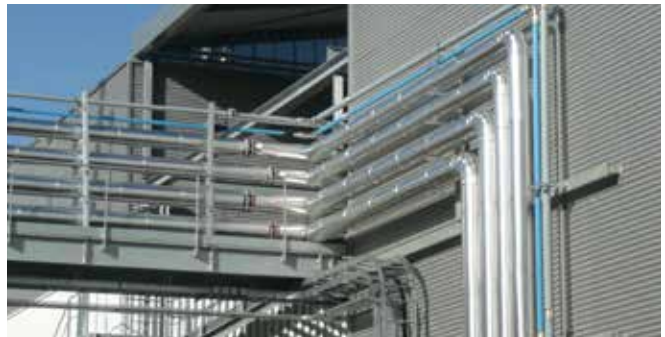
Outdoor installation Transair® 6" (168 mm)
