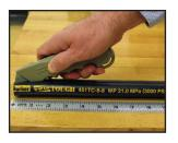
B.) To start the cut, place the blade in the center of that valley (web) drawing the knife with constant pressure.
