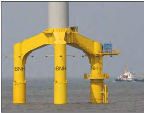
▲ Offshore wind turbine leveling: Enerpac's synchronous lifting system was the solution for leveling support cross pieces on 80 wind turbines.
