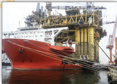
Synchronous superlift and launch
