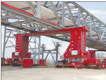
▼ Lifting an oil and gas pipe module
