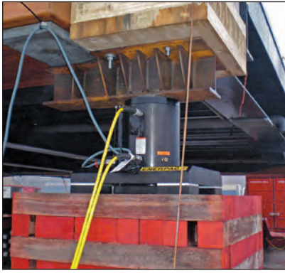
◀ Typical stage-lift application using a custom built Enerpac system to lift the 360 ton Akkerwinde wooden bridge in the Netherlands.
